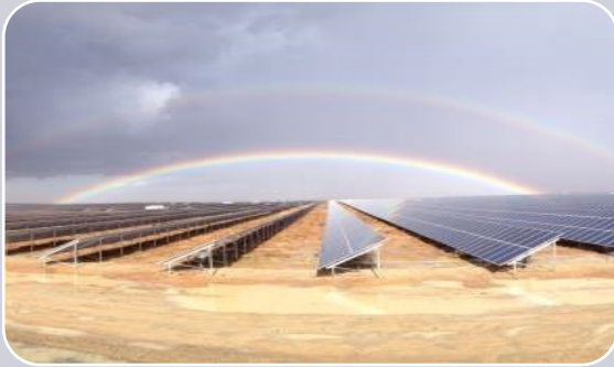
UTILITY SCALE PV
